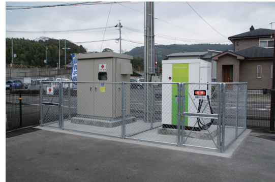
Fig. 4 The charger for the South Korean HFG electric bus does not use CHAdeMO
